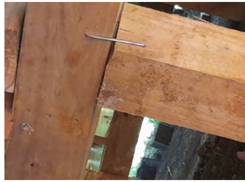
Ordinary pile screw nail is required to NZ S3604. Fixings above also required
