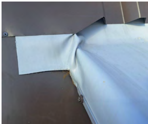
Membrane in contact with metal roof
