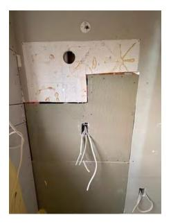
[18] The following photographs of the plaster board under the waterproofing membrane were taken when remedial work was undertaken.
